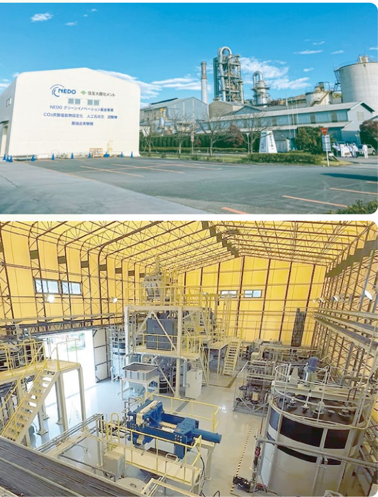
Exterior and interior views of the pilot-scale recycled CO 2 artificial limestone manufacturing test facility at the Tochigi Plant
