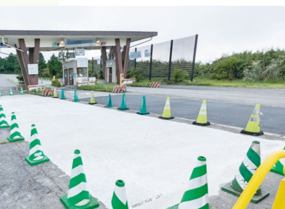
Roadway using next-generation low-carbon semi-flexible pavement
