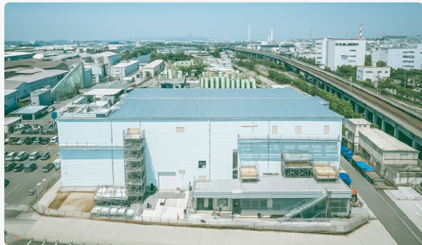
New electrostatic chucks manufacturing building under construction (Ichikawa City, Chiba Prefecture)
