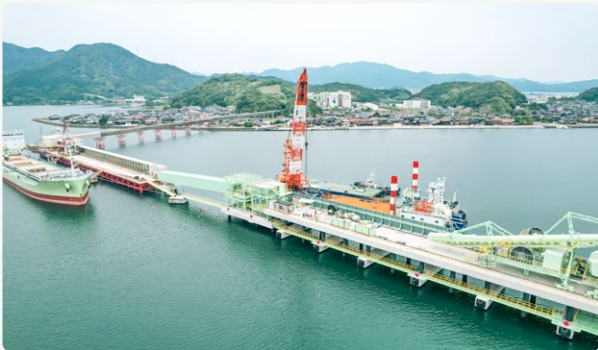
Extension work on the shipping berth at Senzaki Port (Nagato City, Yamaguchi Prefecture)
