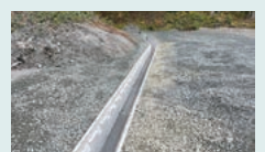
U-shaped groove installed at the site of the direct control project
