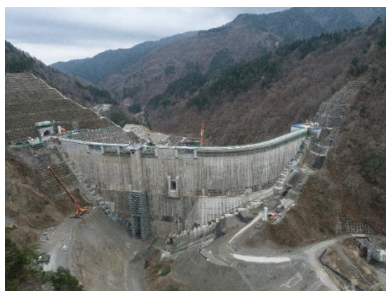
Uchigatani Dam (Gujo City, Gifu Prefecture)
