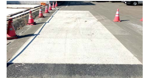
Next-generation low-carbon semi-flexible pavement after use
