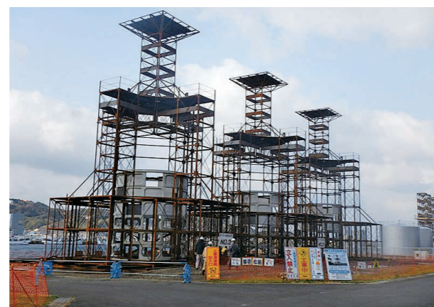
Hybrid Artificial Marine Reef Super SK1300S ready for installation in water
