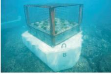
The K-hat Reef Beta, a concrete block with seaweed planted on it and covered with a net right after nstallation in water
