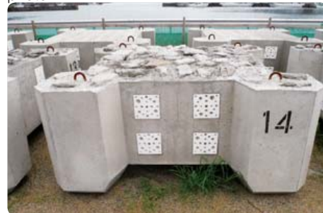
Example of an artificial reef for lobsters using Ebikuru House
