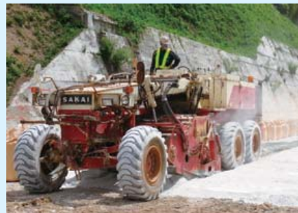
MAGICAL FIX ® being spread using the adsorption method
