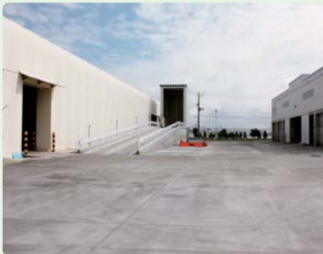
Hachinohe Port Waste Warehouse of Hachinohe Cement Co., Ltd.
