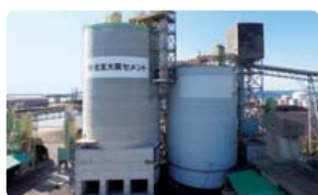
Onahama Service Station (Iwaki City, Fukushima Prefecture)
