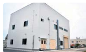
New building (Ichikawa Office, Chiba Prefecture)
