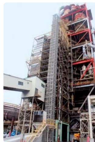
ASR inserting equipment in Ako Plant
