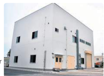
New building (Ichikawa Office, Chiba Prefecture)
