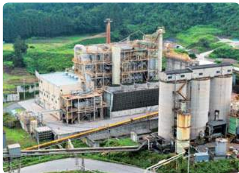
Tochigi Plant biomass power generation facilities
