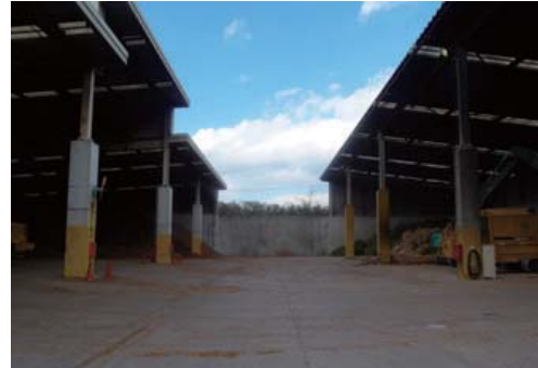
Wood waste storage warehouse at the Kochi Plant
