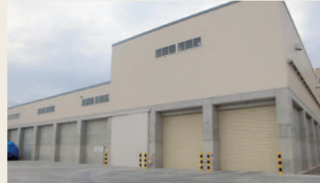
Facilities at the Hachinohe Port for sorting ordinary incinerator ash
