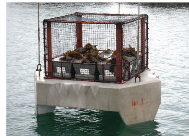
Submerging the K-hat Reef Beta multifunctional seaweed cultivation artificial marine reef (with Ebikuru House)
