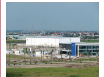
Manufacturing plant (SOC VIETNAM, Hung Yen Province, Vietnam)
